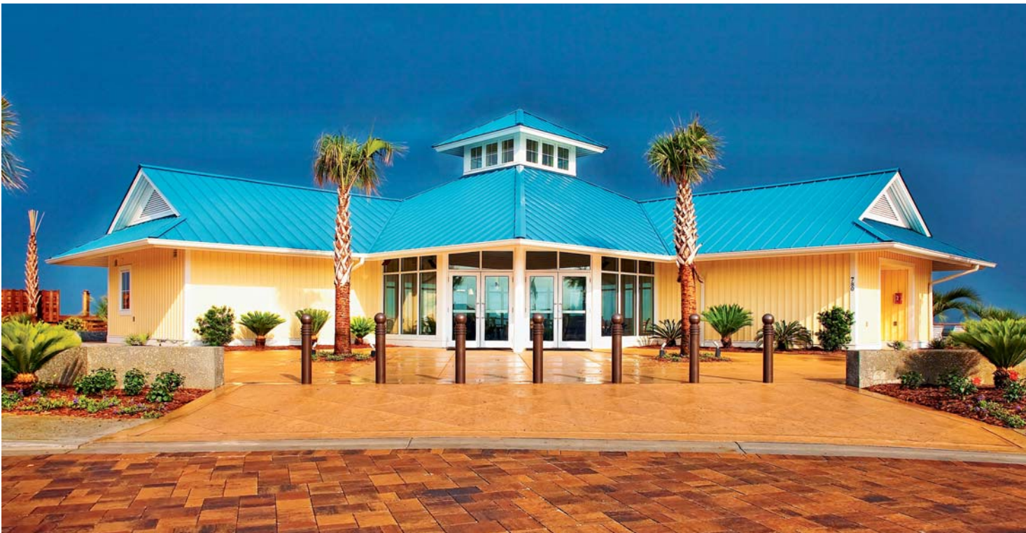
BEC Construction has completed several commercial projects and Berry took great pleasure in building the Litchfield By The Sea Clubhouse. The blue standing seam metal roof and yellow board and batten siding make this clubhouse stand out from the surrounding buildings on the oceanfront.
